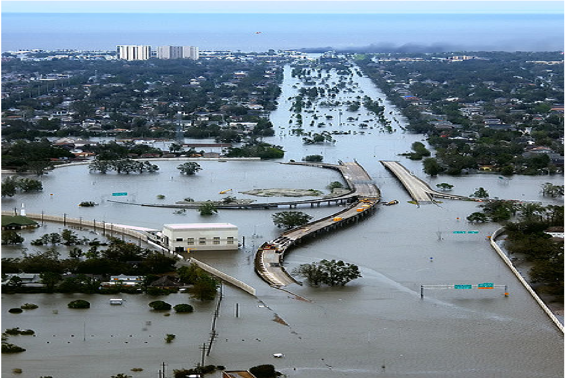
Flooded I-10/I-610/West End Blvd interchange and surrounding area of northwest New Orleans and Metairie, Louisiana
